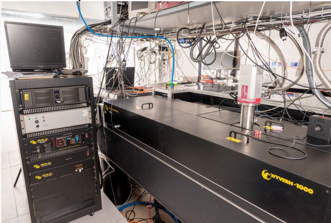
Complete beam enclosure
